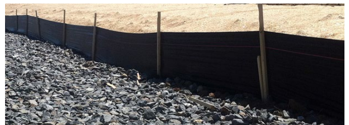
An example of silt fencing and rubble
