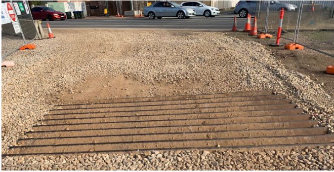
Example of a rumble grid and rubble at an exit gate
