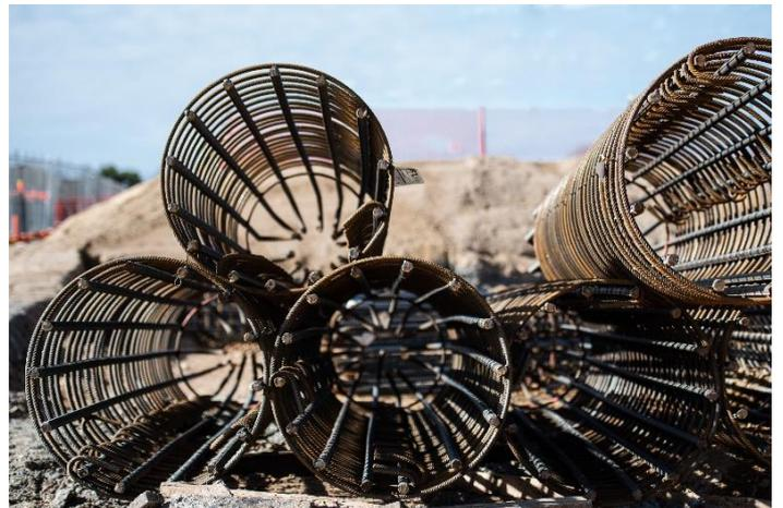
*The steel reinforced cage that is placed into the pile*
