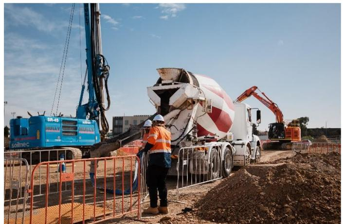
*Concrete being poured into the pile*
