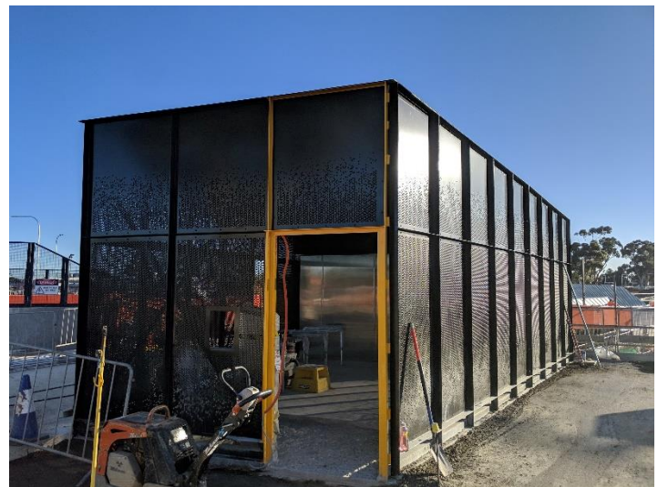
Construction of the amenities building, looking east
